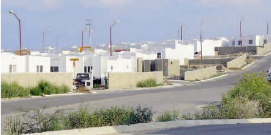
Figure 13: Neighborhoods like this working class neighborhood in northern Mexico have grown largely as a result of INFONAVIT, which constitutes over half of the mortgage market in Mexico. Photo © Brendan McBride. Source: https://unhabitat.org/sites/default/files/download-manager-files/Affordable%20land%20and%20housing%20in%20Latin%20America%20and%20the%20Caribbean.pdf
